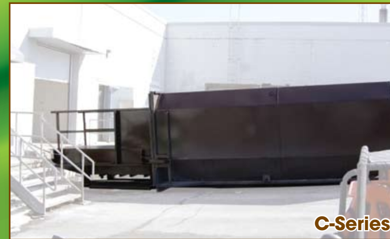
Walk-on Deck with Safety Railing
